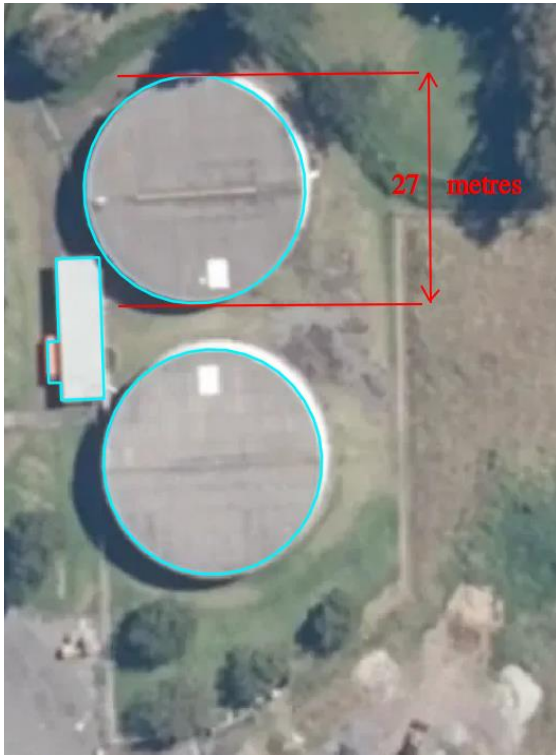
Correct capture of two circular tanks with each diameter greater than 5m, or each area greater than 20m 2 .
